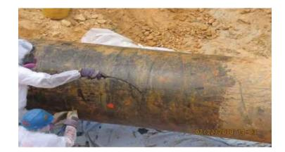
Winter Environmental was selected to provide on-call asbestos abatement services for Dixie Pipeline Company. Abatement services were performed along sections of the natural gas pipeline where engineering and construction crews were conducting regulatory mandated integrity testing. The pipeline systems measured up to 60 ft in length and six to 18 inches in diameter at multiple locations throughout the network system.
