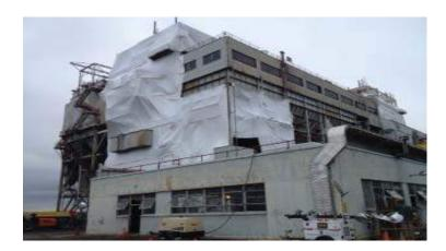
Winter Environmental performed asbestos abatement and selective dismantling of the Duke Energy– Lee Power Plant located in Goldsboro, North Carolina. This 382 MW power plant, maintained three coal fired boilers, associated turbine buildings and decks, precipitators, administration and contractor buildings, and other ancillary buildings on site that required abatement.
