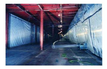
Winter Environmental provided asbestos abatement and interior demolition services to six floors in this occupied, eight-story, Class A office building located in Atlanta, GA. This challenging project also involved working around the tenant-occupied first and fifth floors and abatement of the elevator shaft on weekends in order to maintain elevator access to the occupied floors during normal business hours.
