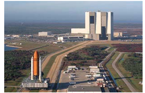
In 2014, the National Aeronautics and Space Administration (NASA), called on Winter Environmental to perform Asbestos Abatement on towers B and D of the Kennedy Space Center Vehicle Assembly Building, and Asbestos Abatement on the Maintenance & Operations Buildings.
