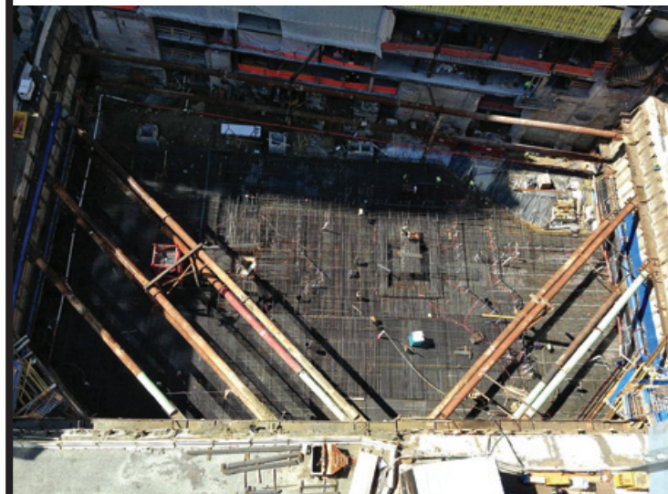
J Derenzo Cos. (No. 167) excavated 36 ft below grade in preparation for the single-largest concrete pour in Boston history—by S&F Concrete (No. 150)—for the 60-story, 1.1-million-sq-ft, mixed-use Millennium Tower.
