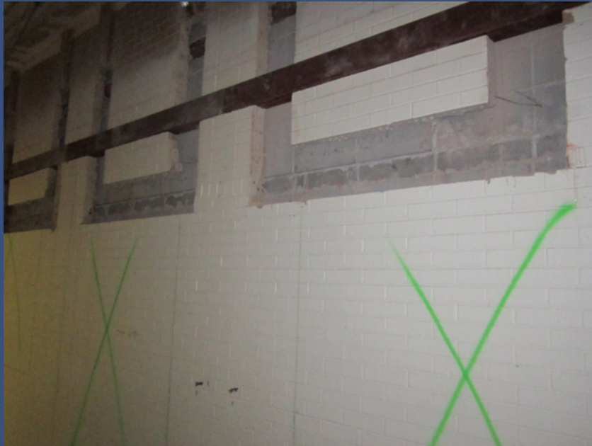
Area of southern hallway following abatement of PCB containing caulk.
