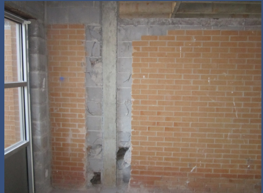
Area of southern portion of the building following abatement of PCB containing caulk.
