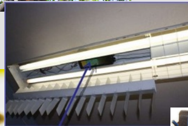
PCB-containing Ballast
